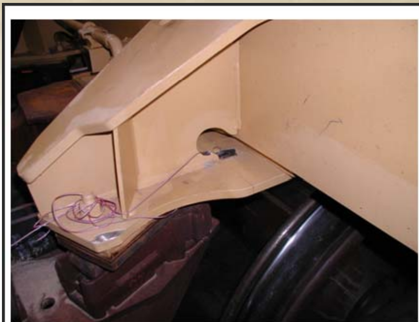
Typical Strain Gage Installation on Side Bearing Bracket
